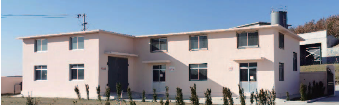
壓縮空氣及配電樓
